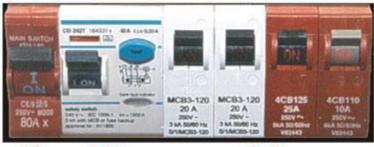
Main Switch Safety Switch Circuit Breakers **Typical switchboard** – this shows the main switch, safety switch with test button, and four circuit breakers.
